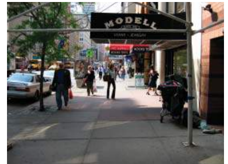
Cantilevered awnings supply promotion and shaded cover without additional sidewalk clutter. Shown: 23rd Street between Lexington & 3rd Avenues.
