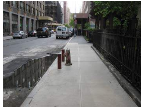
Standing water in gutters is unsanitary and, at crosswalks, reduces the comfort of accessibility.
