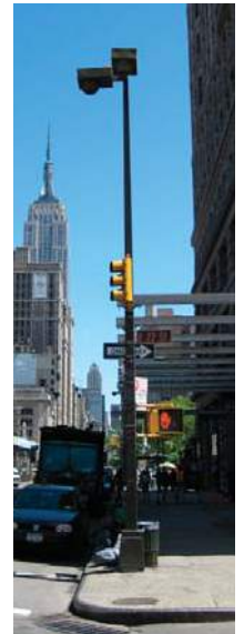
Fifth Avenue 1970's Pole
