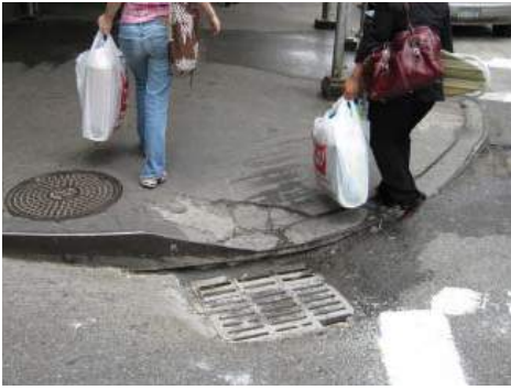
Failing catch basins at corner intersections erode curbs & curb cuts, and affect accessibility. Shown: Broadway between 21st & 22nd Streets.
